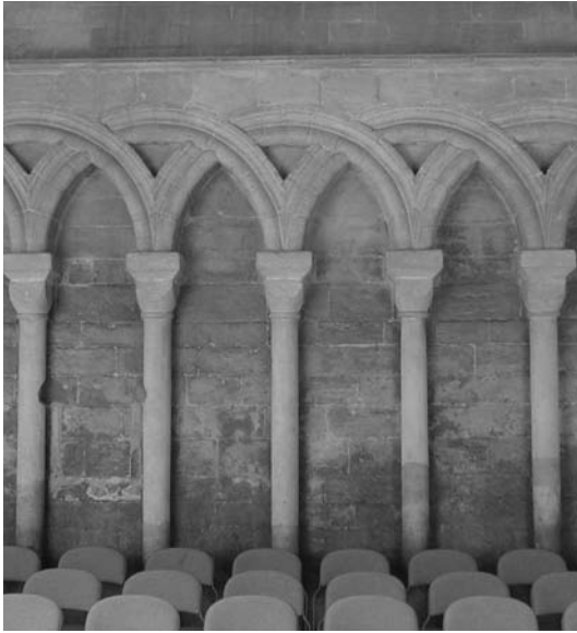
Part of the southern wall inside Peterborough Cathedral. The Vesica Piscis link is clearly defined.
